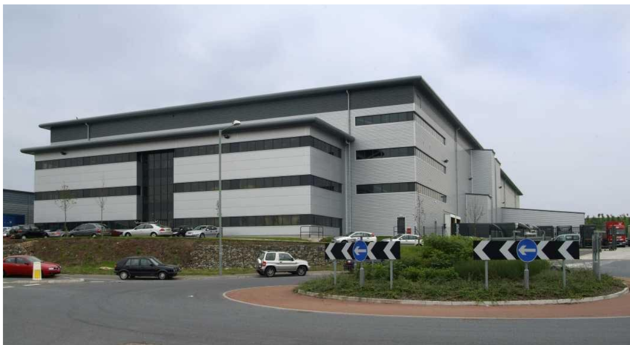
Grahams' new integrated distribution, warehousing and head office site at Matrix Park
